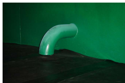
Figure 8. The inlet pipe elbow of the demineralized water storage tank (the overlooked photo) 图 8. 除盐水储水箱进水管弯头(俯视照片)
