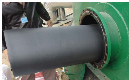
Figure 5. Raw materials of the floating roof put in the demineralized water storage tank from lower part of the tank manhole 图 5. 浮顶原材料由水箱下部人孔放入水箱内部
