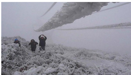
Figure 1. Zhaotong transmission line icing ( >20 mm)
