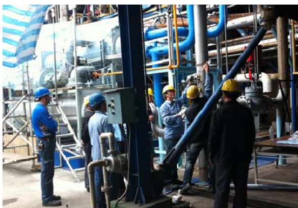
Figure 6. Hot water inlet being equipped 图 6. 热水进口管配置时的情形
